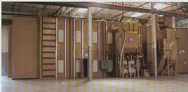
Turnkey Blast Room Installation
